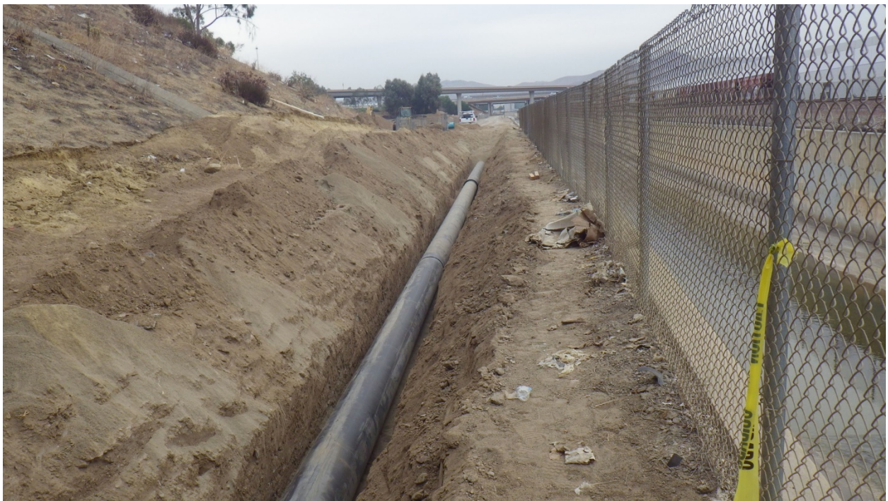
Figure 3: Section of pipeline realigned to minimize bends and elevation changes.
