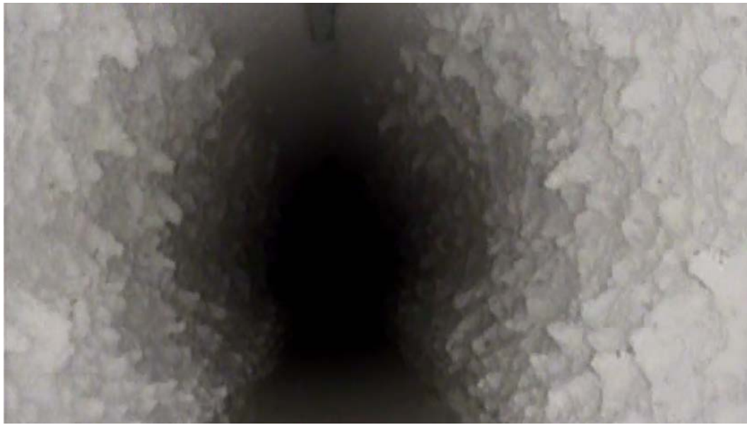
Figure 4: Section of heavily scaled pipe prior to cleaning.
